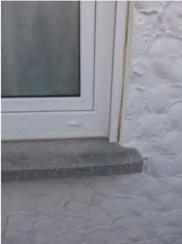
25 a Detail Fenster
