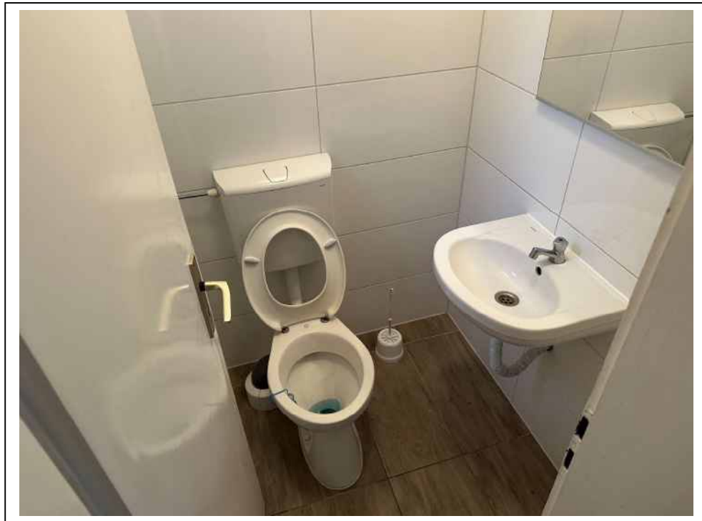
Foto 11: Blick in das EG-WC
