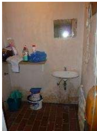
Blick in Abstellraum
