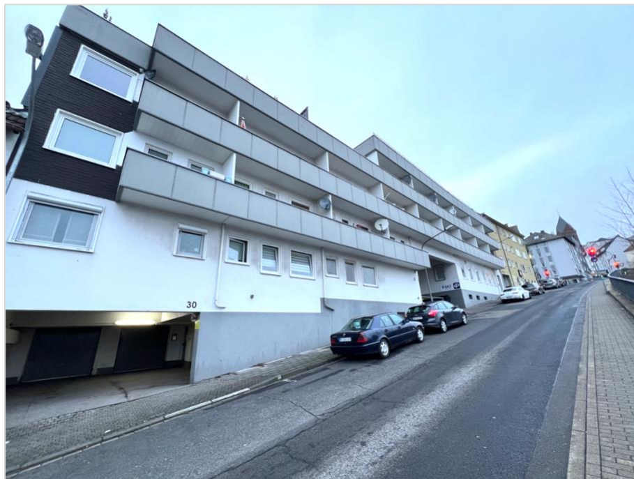
WET-Anlage Papenberger Str. 26, 28, 30
