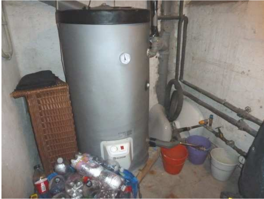
Warmwasserboiler
